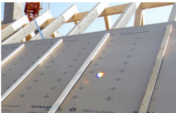
Figure 3: Subroof with increased requirements (rain tight according to ZVDH)
